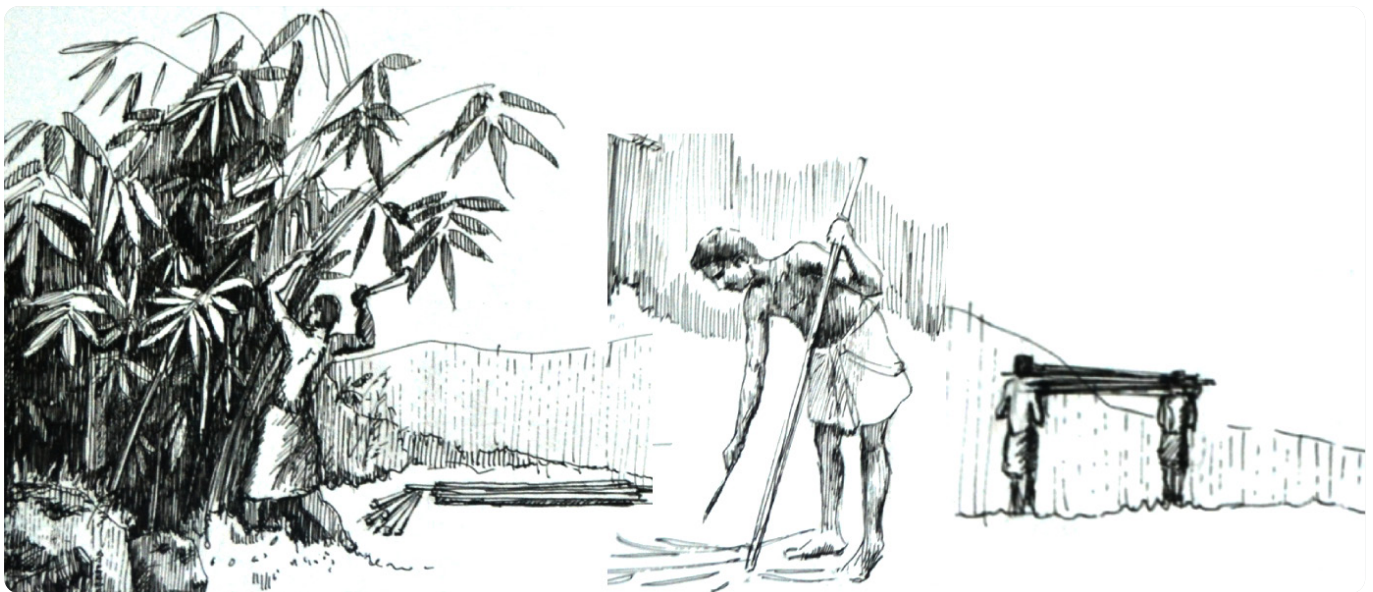
4. Eeta with relatively straight sections throughout its length are selected and the outer-most layer, comprising largely of foliage, is peeled off. They are cut into desired length, tied in a bunch, and carried onto the site.
